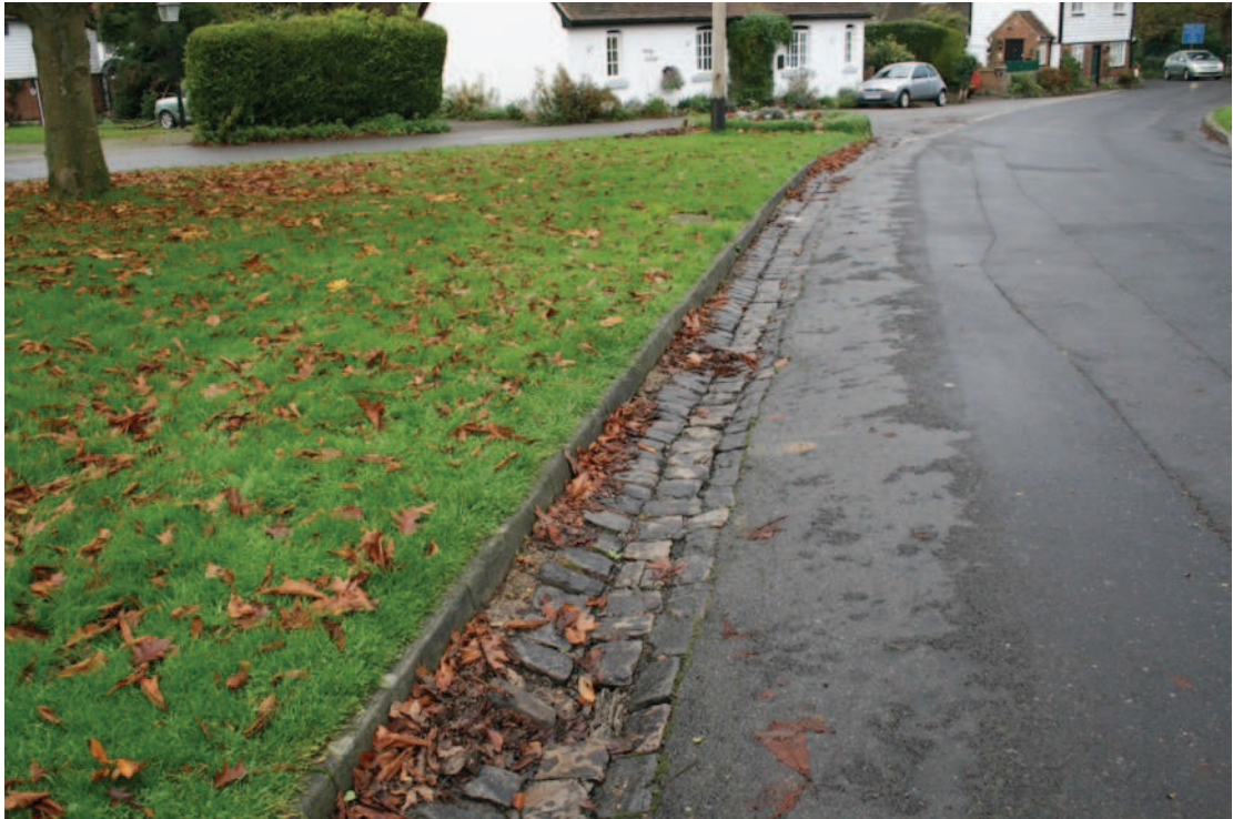
Figure 11: Ragstone gutter, Boughton Green
