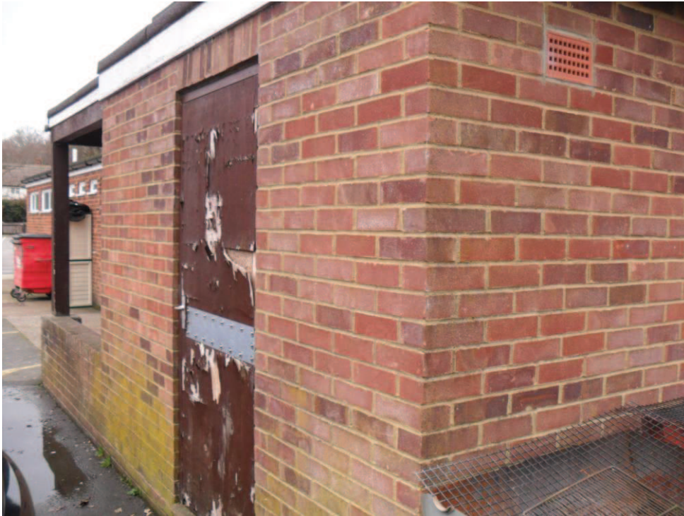
Photo no 5227 External Joinery to Club House - Weathered, use worn and defective
