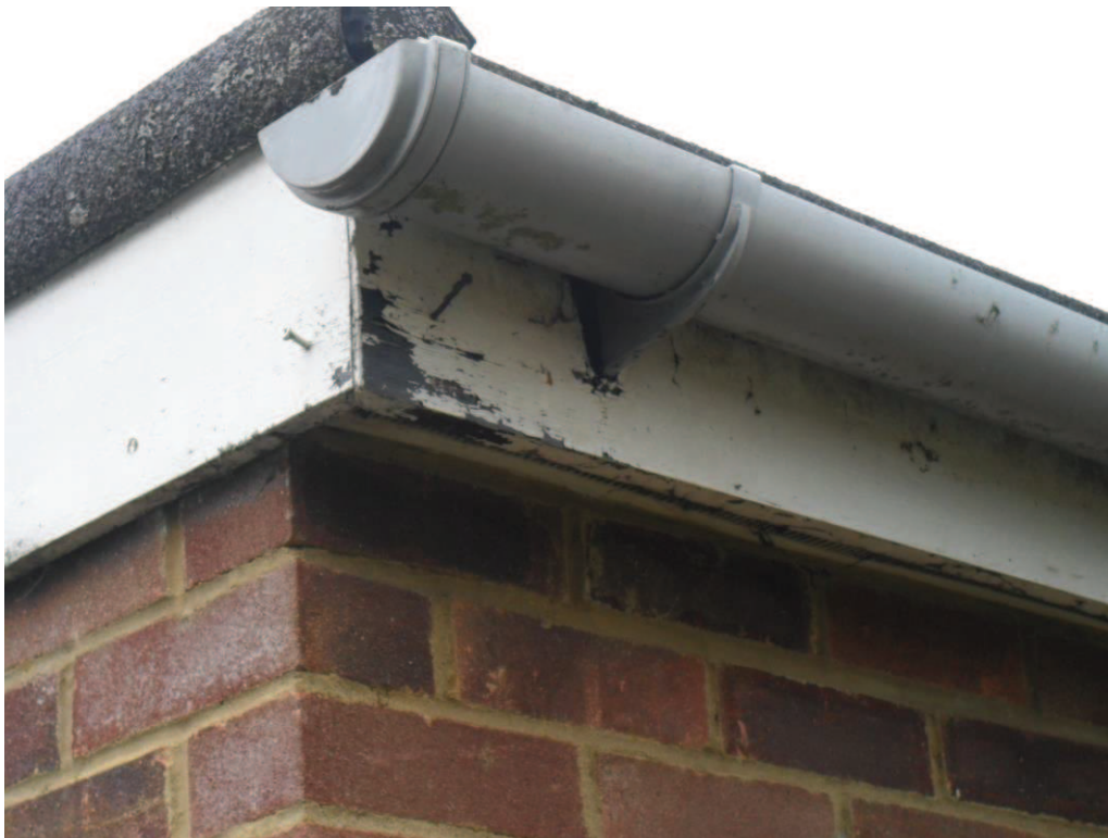
Photo no 5228 External Joinery to Club House - Weathered, use worn and defective
