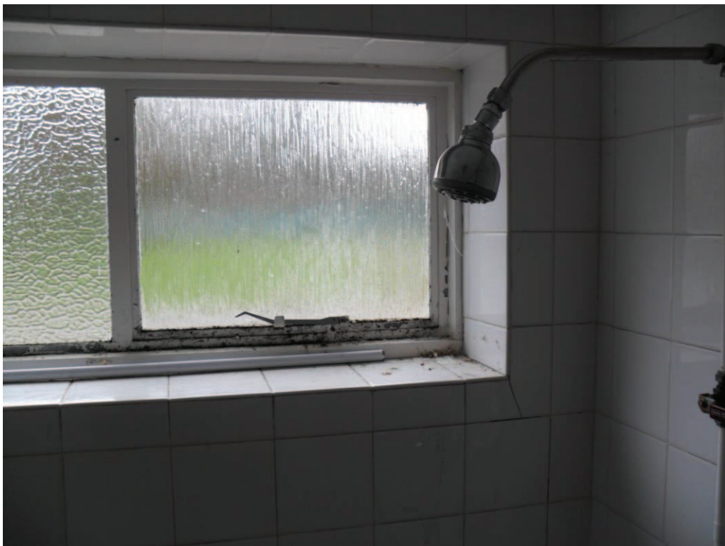
Photo no 5210 Defective metal window frame and age worn insanitary Shower
