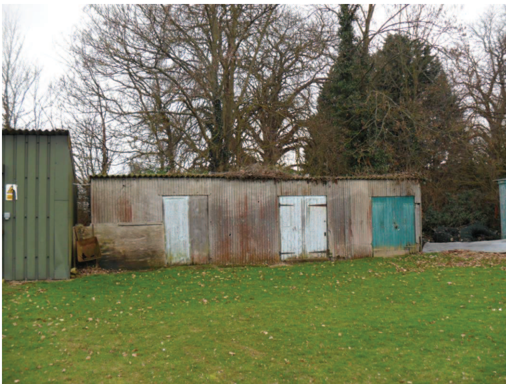
Photo 5200 Asbestos cement sports storage building- Dilapidated – To be removed
