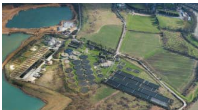
Aylesford Wastewater Treatment Works
