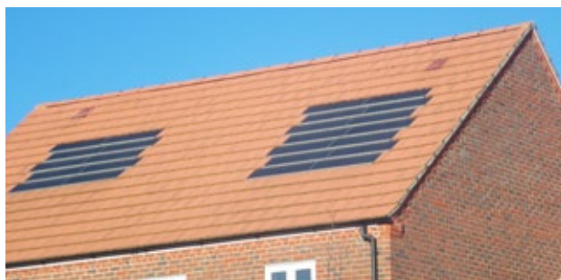
Recent development in North Loose with PV panels replacing tiles
